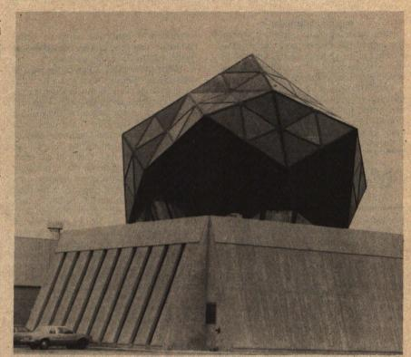
This geodesic dome is located in the neutrino area of the laboratory. It is constructed of discarded cans sandwiched between polyester-reinforced fiber glass. The dome contains 120,000 cans, which were donated by the public. (photo by Phil Karch)
